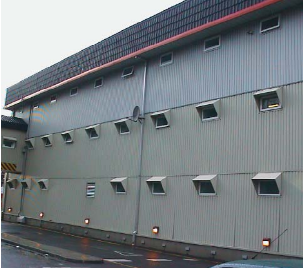
LESSONS LEARNED Colombian police station design features double-skinned walls to allow defenders to move under cover.
